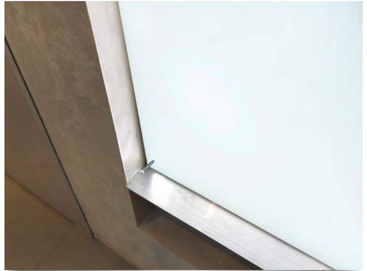
**PLEASE NOTE:** If screws cannot be used on the artistic surface, the DAKOTA SEAMLESS panels must be secured directly to the wall using screws at the panel corners.
